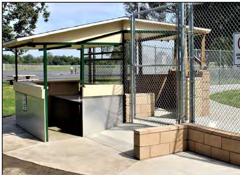
The timing shelter has a new equipment ramp and eight-foot gate.
