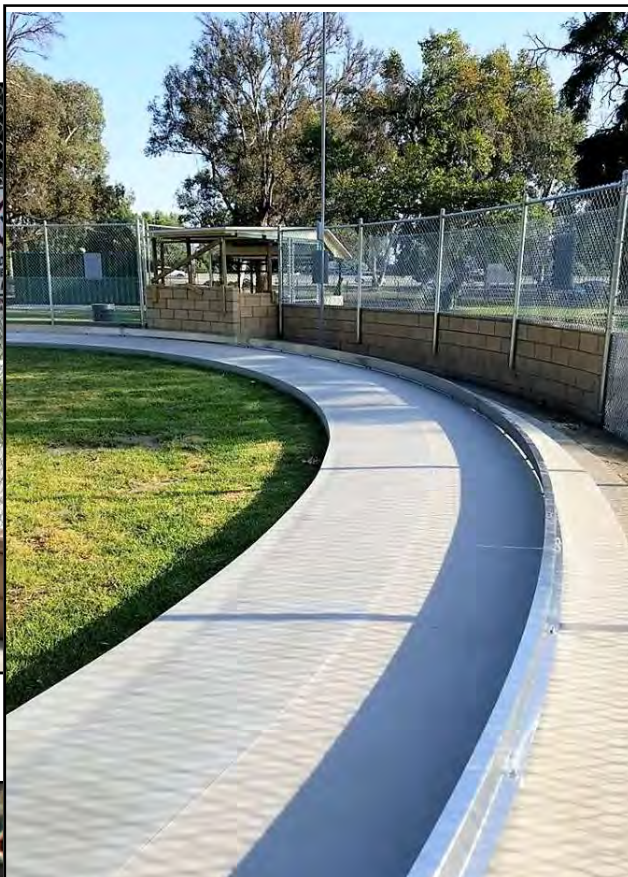
The track has a new stainless steel guard rail.
