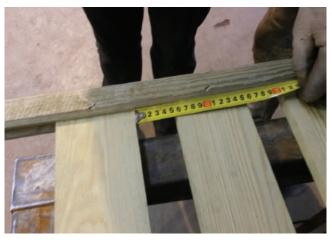
**Step 7**Fix the new beams using staples (battery or pneumatic) or screws for wood.
