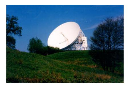
The Mark 1 telescope, operational in 1957, was upgraded to Mark 1A in 1970 / 71 and renamed the Lovell Radio Telescope in 1987. Height 89 metres, diameter of bowl 76 metres, weight of bowl 1,500 tonnes. It is a Grade I listed building.
