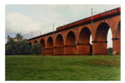
The Viaduct has 23 arches, each 90 feet high and with a span of 63 feet. It was built by the Manchester & Birmingham Railway Company. Eight lives were lost during its construction, which was completed in 1842.
