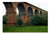
The Viaduct has 23 arches, each 90 feet high and with a span of 63 feet.
