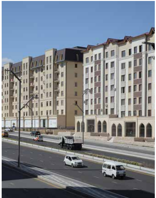
A new modern apartment block being built in Yashnobod. While many of the Soviet era apartment blocks are at most, seven to nine storeys, the new apartments are being built much higher. Overall, these will have much nicer and newer furnishings than Soviet era ones, but the prices will reflect that.
