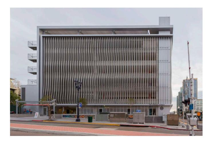
Reminiscent of ripples in the San Diego Bay, the CloudWall™ surface follows the recently completed waterfront park. The facade encompasses the building's seven aboveground levels. Three additional levels exist underground. The panels were installed using custom extruded channel embeds which were set in concrete. Zahner worked with McCarthy to coordinate the location for each embed.
