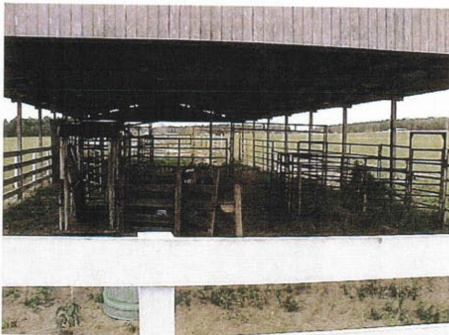
Photograph 18. View of an open pole barn located on the east portion of the subject property
