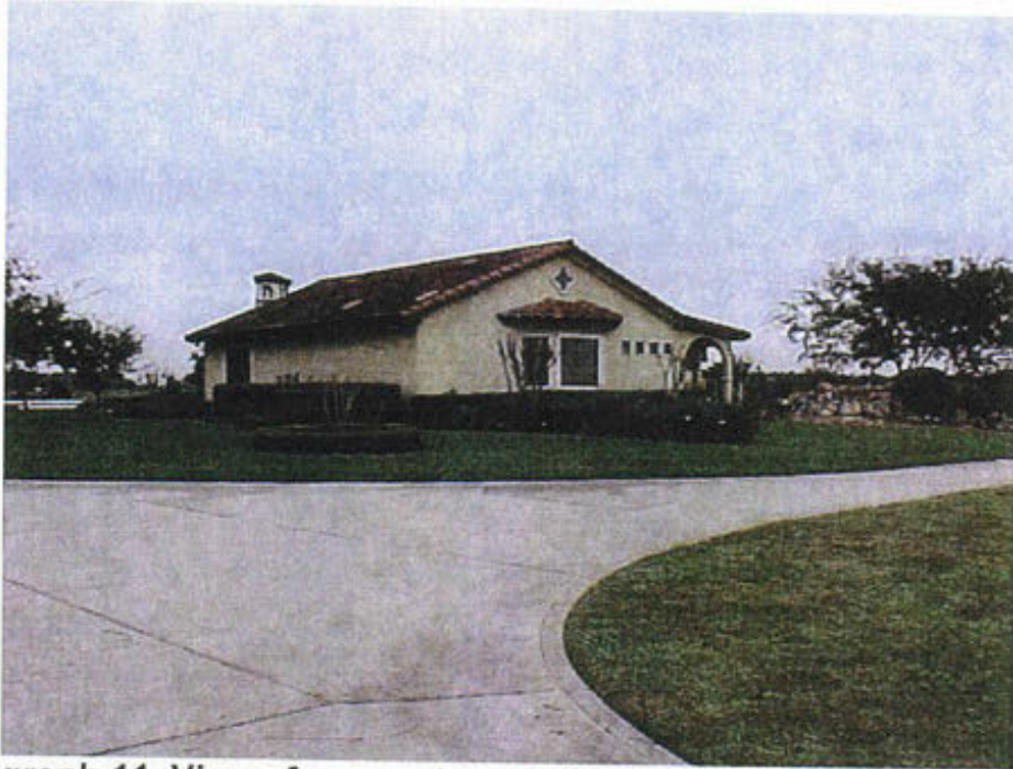
Photograph 11. View of a one-story residence located on the southeast portion of the subject property
