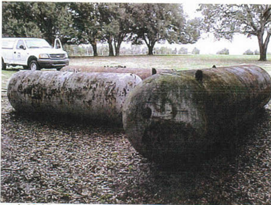
Photograph 22. View of three (3) ASTs, used for no purposes, located on the northeast portion of the subject property
