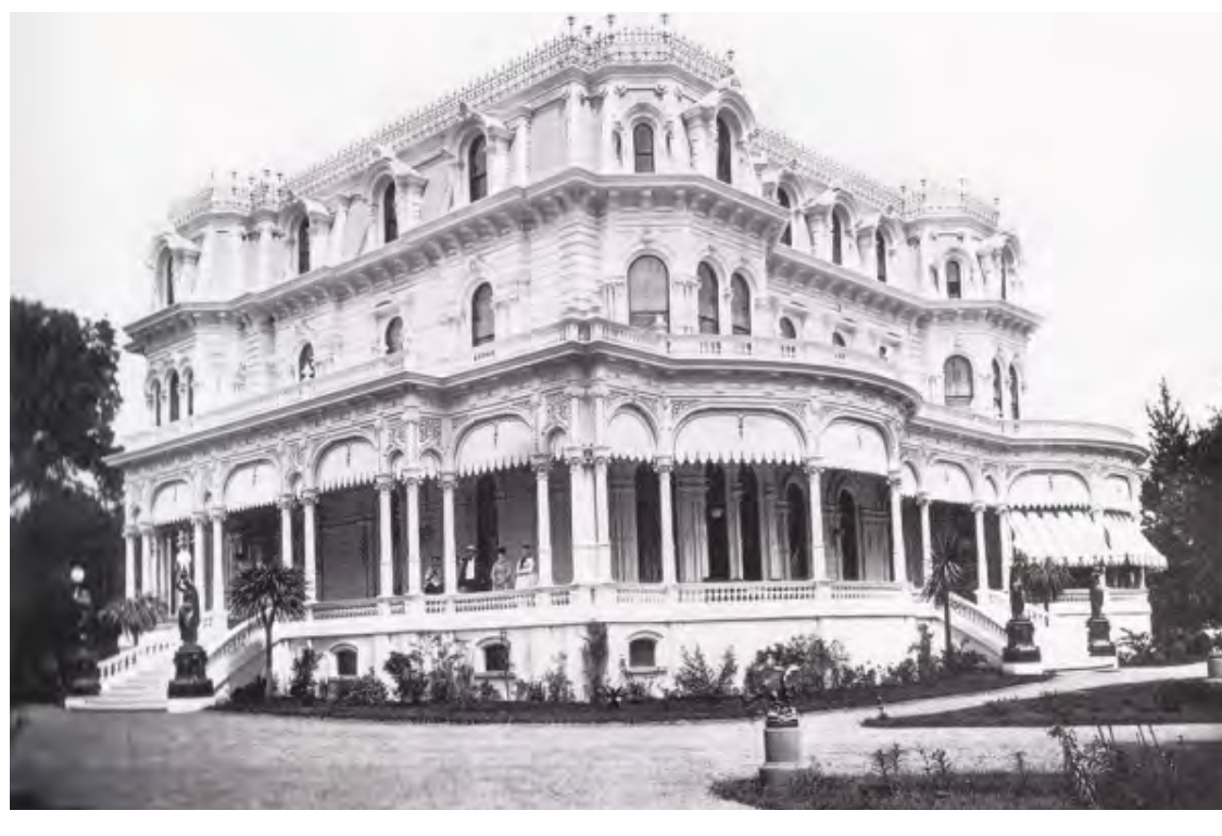
Thurlow Lodge/Sherwood Hall
