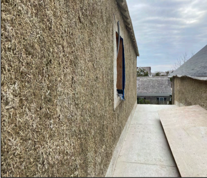
Image #4 - Connector walls insulated
