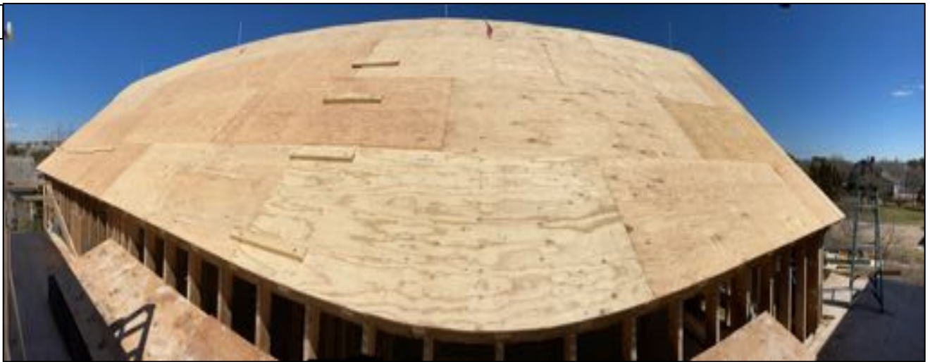
Image #8 - Plywood complete on south roof of the North building
