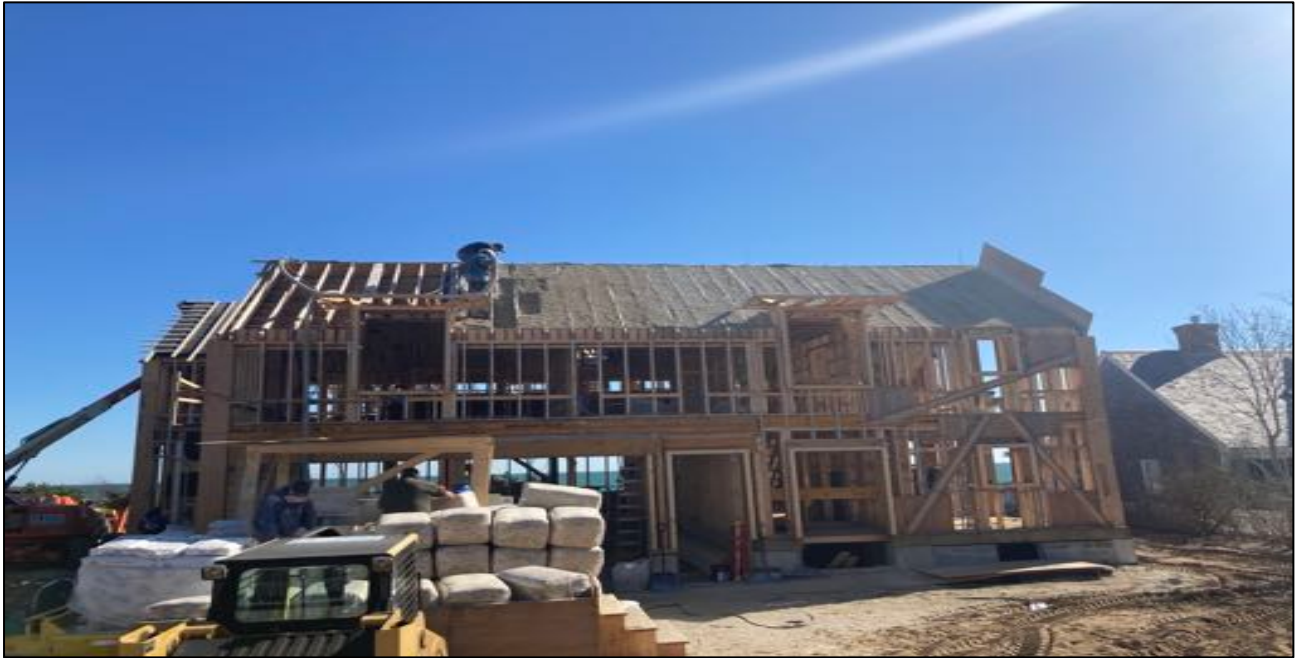
Image #1- Solitex and sleepers going on the roof
