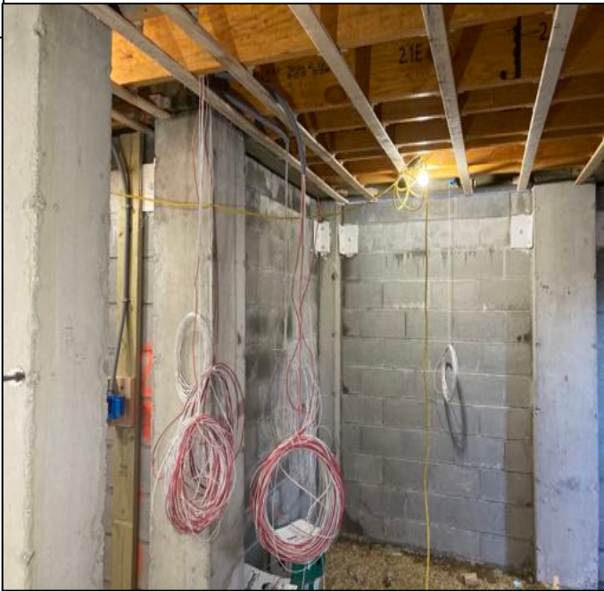
Image #4 - Wire being dropped to basement
