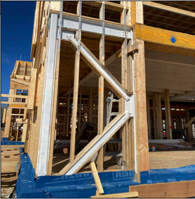
Image #4- Moment frame receives epoxy for hemp lime
