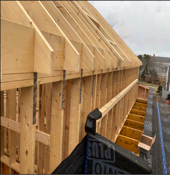
Image #4 - SS strapping nearly completed around building
