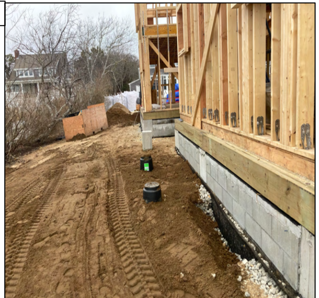
Image #3 - Piers in place for west side deck. When poured the forms will be square from sub grade up
