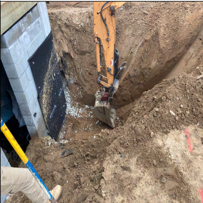
Image #7 - Digging complete for egress forms
