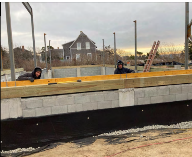
Image #3- Packed out steel beam
