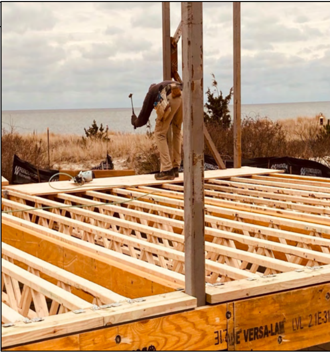
Image #4- 14" Triform joist installation
