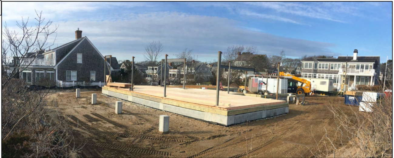
Image #9 - Aggregate added and foundation backfilled. Still have some add work to do in the garage
