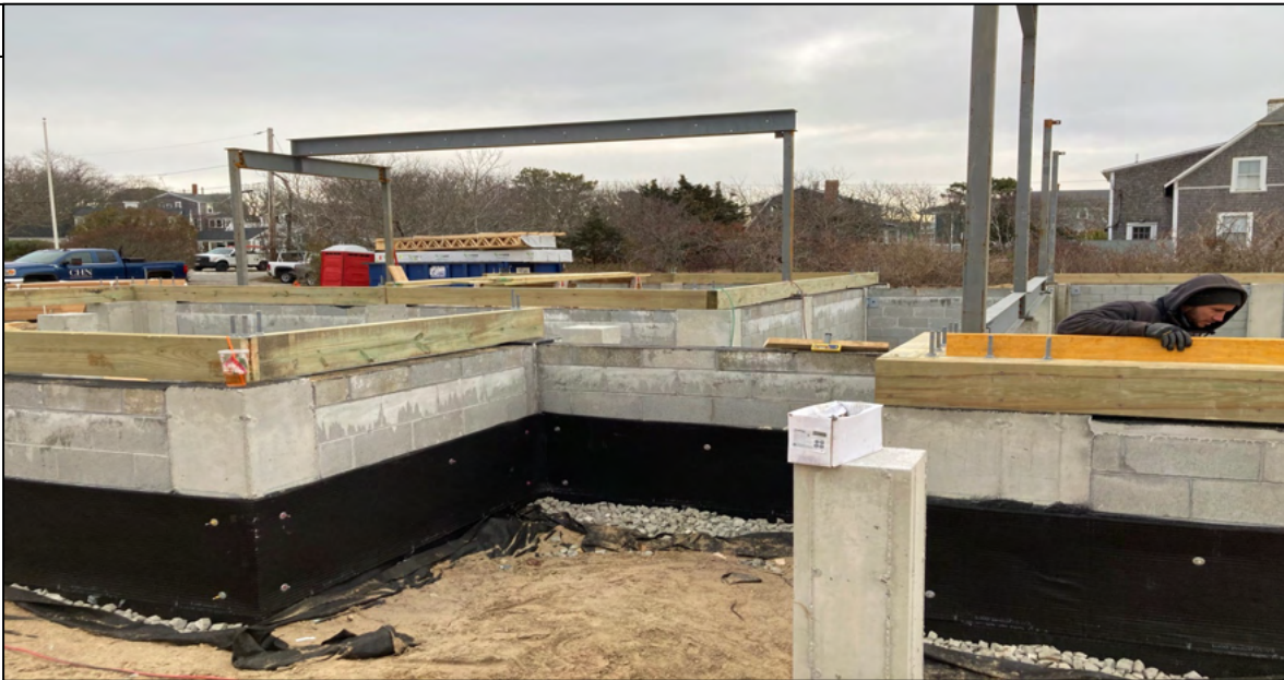
Image #1- Sill plates being installed
