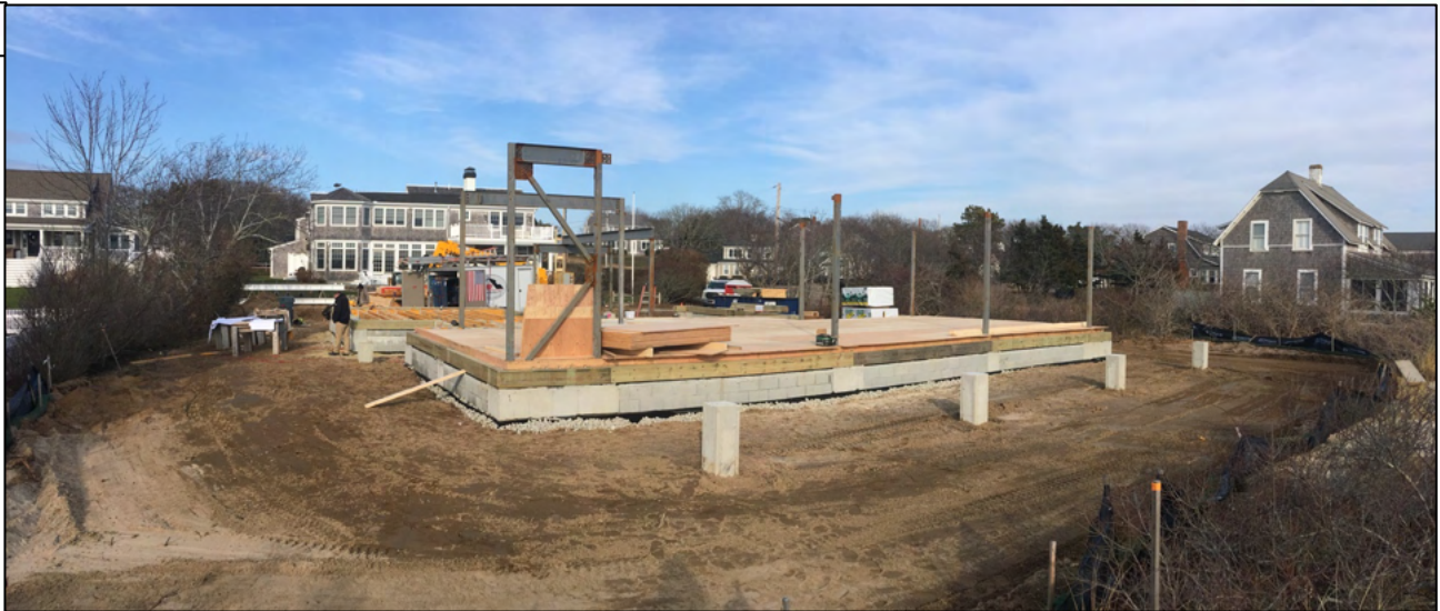
Image #8 - Aggregate added and foundation backfilled
