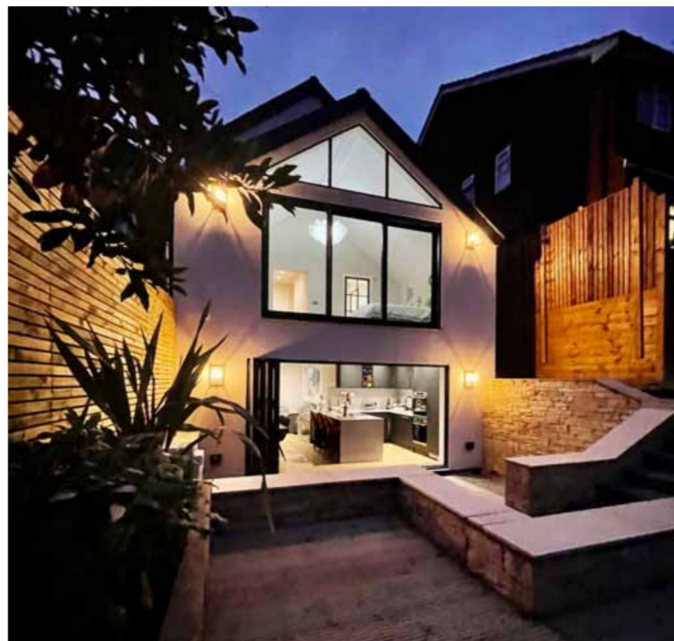
External shots of the new rear extension
