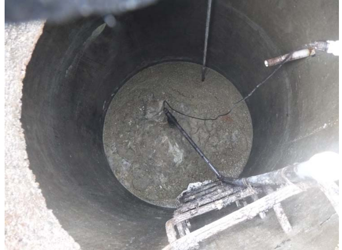
PRE-TRIAL: ONE MONTH FOG BUILDUP 1/25/2017
