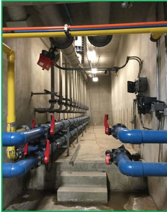
Before Example of 1 of 5 membrane tank pipe galleries
