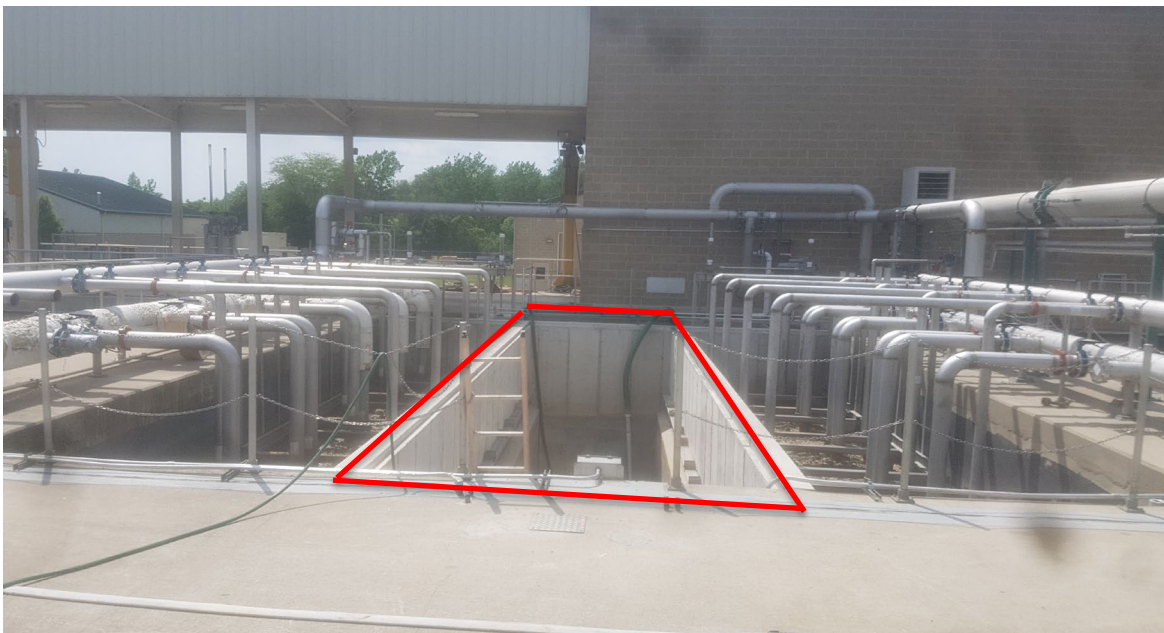
Figure 4 – FibrePlate Membrane Tank at Delphos – Train 2 in the center being installed
