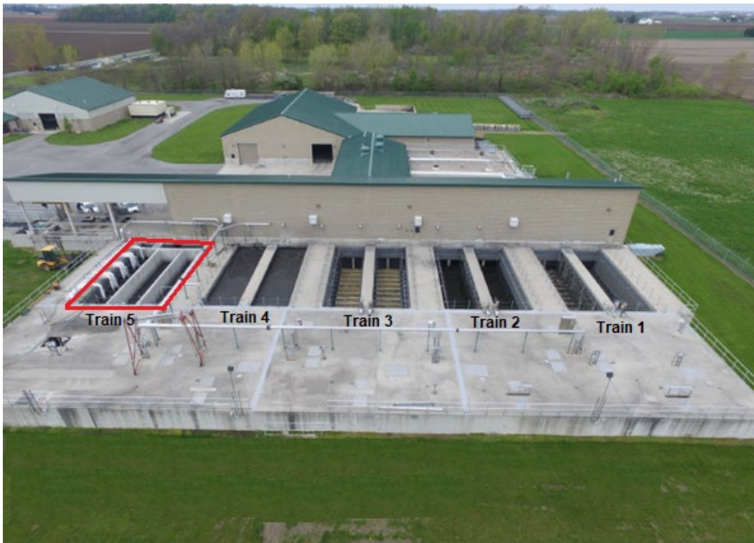
Figure 3.0 – Delphos aerial view of membrane tanks with Train 5 retrofit
