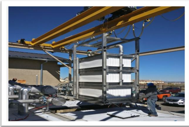
Installing FibrePlate™ cassette in one of the 2 membrane tanks using the overhead crane.
