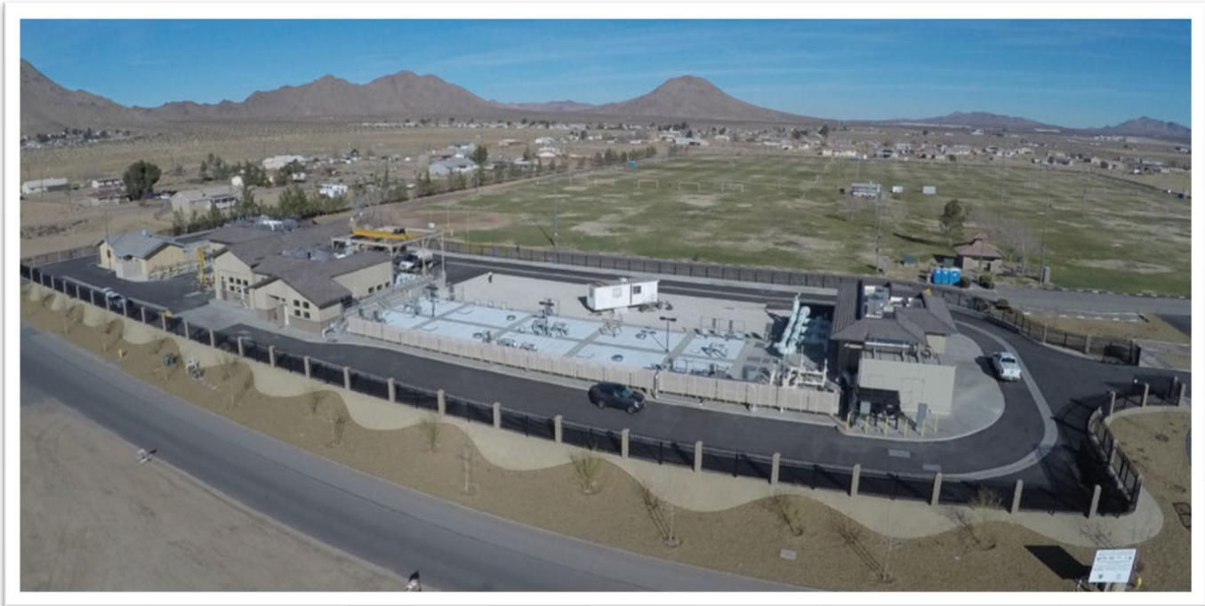
In 2014, the Victor Valley Wastewater Reclamation Authority, in California’s Antelope Valley northeast of Los Angeles, selected FibrePlate™ membranes for two new, decentralized wastewater reuse scalping plants. The sister membrane bioreactor (MBR) plants were designed by Carollo Engineers to treat and reuse the wastewater locally instead of pumping it twice, to and from the main regional plant. These plants were built to enable future development and regional growth.
