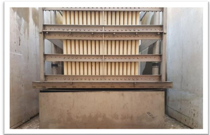
At 1 MGD, the 2 FibrePlate™ cassettes only occupy half the space in the membrane tank. Each tank has room for 2 more cassettes which will double design flow to 2 MGD without additional construction costs.
