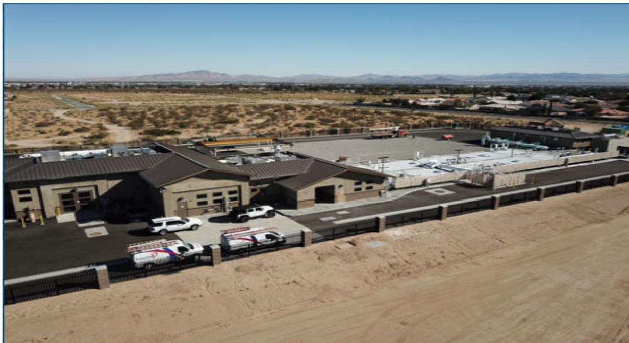
2014, the Victor Valley Wastewater Reclamation Authority, in California’s Antelope Valley northeast of Los Angeles, selected FibrePlate™ membranes for two new, decentralized wastewater reuse scalping plants. The sister membrane bioreactor (MBR) plants were designed by Carollo Engineers to treat and reuse the wastewater locally instead of pumping it twice, to and from the main regional plant. These plants were built to enable future development and regional growth.
