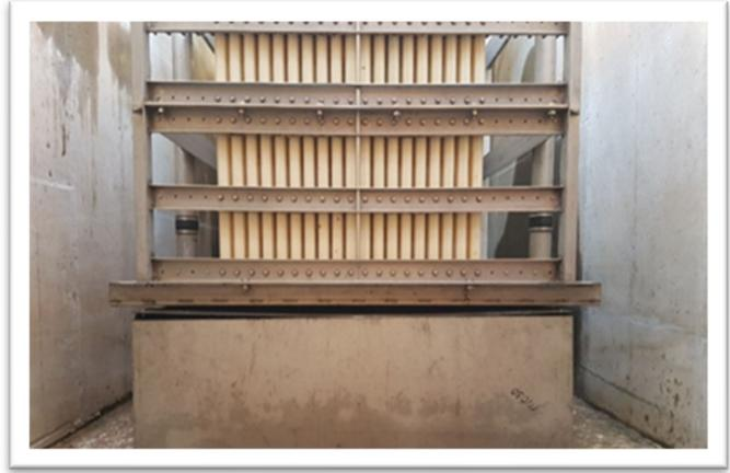
At 1.5 MGD, the 2 FibrePlate™ cassettes only occupies 2/3 of the space in the membrane tanks. The tanks can be equipped with 2 more cassettes, allowing to increase the flow to 2 MGD without additional construction costs.
