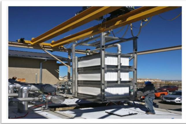
FibrePlate™ cassette installed in one of the 2 membrane tanks, using the overhead crane.
