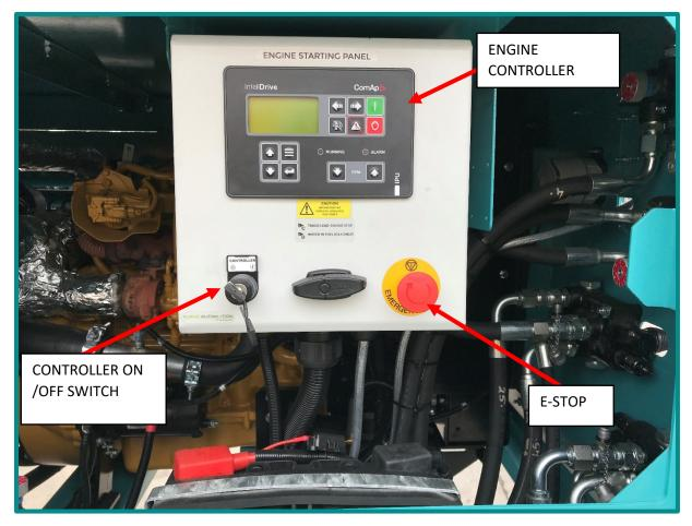
Start the engine by turning the key clockwise to the 1. position.
