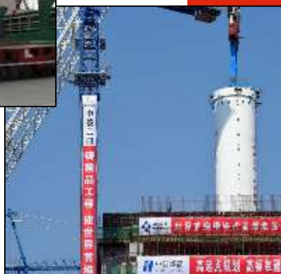
Pressure Vessel Delivery & Installation
