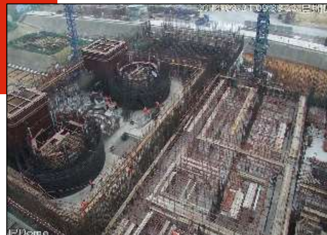
HTR-PM Construction Site
