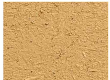
Structure of a well-prepared surface of clay undercoat plaster
