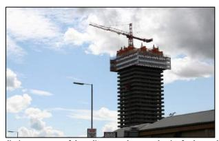
The use of a vertical descending cap as a safety innovation is remarkable and as the version, Top Down Way<sup>TM</sup> developed by Despe<sup>10</sup> is capable of covering three floors so nuisance factors such as dust are contained within the frame and do not escape.
