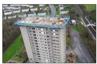
The substitution of the traditional scaffolding wrapping around the structure with that of a mast climbing work platform is while controversial, very interesting as it is considerably faster to install than scaffold and as such may be more desirable from a commercial viewpoint.
