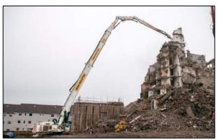
For the purpose of this section, it should be noted that there is no distinction between high-reach and super-high-reach demolition rigs. This is due to the fact that while there is a distinct difference in the movement of the rig and the skill of the operator, the fundamental principles remain the same for demolitions over the height of thirty meters (30m).
