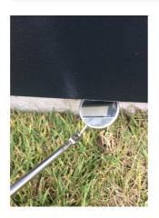
Walls; Does the wall cladding have suitable flashings and damp proof course, and is it free of dampness damage?
