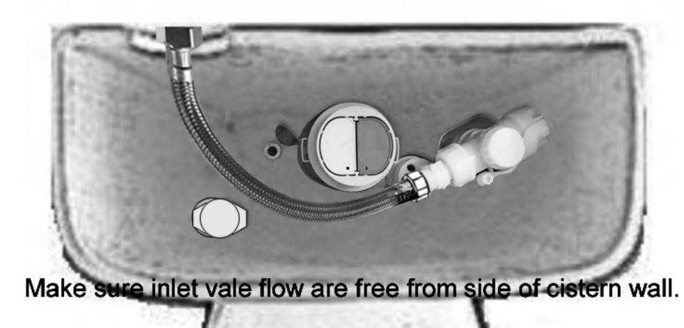
If inlet vale been jam on the cistern wall, it will cause inlet vale keep filling.
