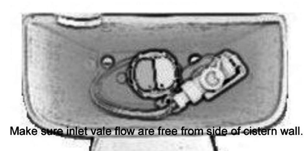
If inlet vale been jam on the cistern wall, it will cause inlet vale keep filling.
