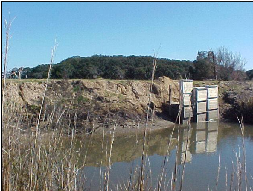
Site of the former bridges at Fenwick Island. The box structures are “stand-pipes,” which control water flow.
