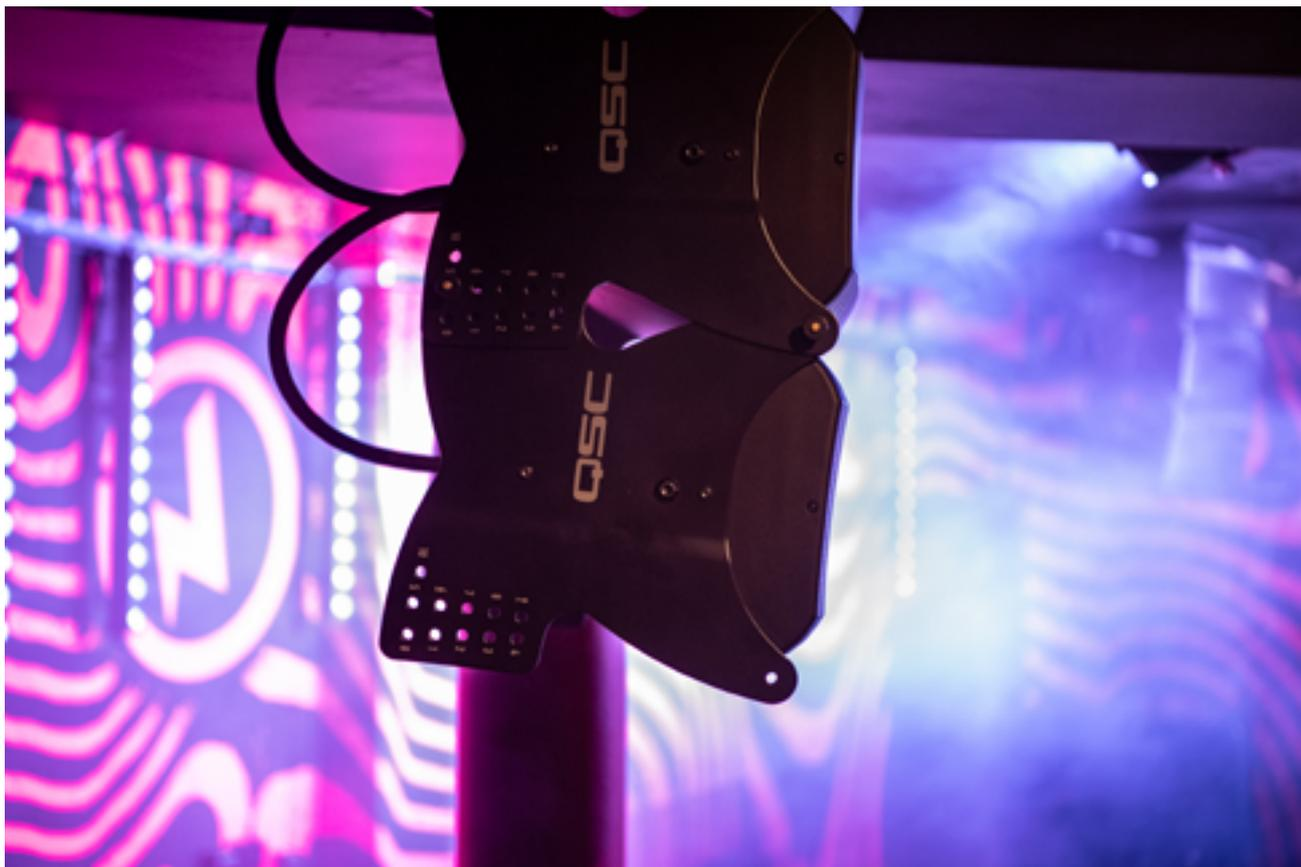
design maximised the power that could be installed in this low-ceiling venue. A Midas M32 mixing console was specified by the client. Adlib also installed a QSC AD-S282H delay loudspeaker to ensure intelligibility was maintained even at the furthest point from which the stage can be seen.
