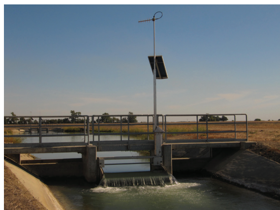
NeuroFlo software controls the actions of the FlumeGates and the flow rate of the pumps to maintain stable water levels.
