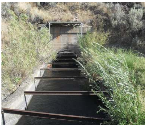
Elevated wood flume
