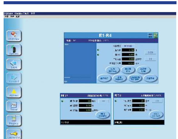
A Chinese language SCADAConnect interface provides operators at Fen River's control centre with real-time flow and water level information
