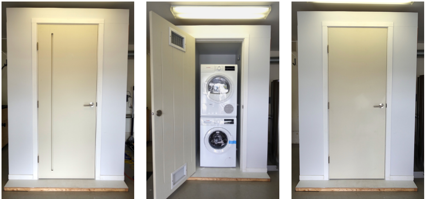
Figure 5 - Test Closet and Samples: VanAir Door, 2 Door Grilles, and Door Without Vents
