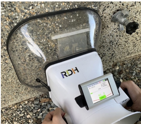
Figure 7 - Flow Hood Measuring Airflow at Dryer Exhaust
