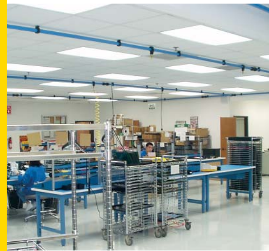
Rigid aluminum calibrated pipe assures clean air and optimum flow rate performance.
