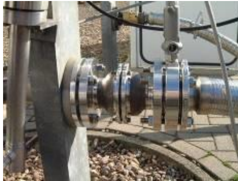
Figure 1 Typical breakaway coupling for liquid filling
