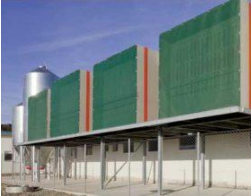
The decentralized system is built to fit Big D's CL wall air inlets but can also be retrofitted for existing wall inlets. Air capacity is 1500 m<sup>3</sup>/hour
