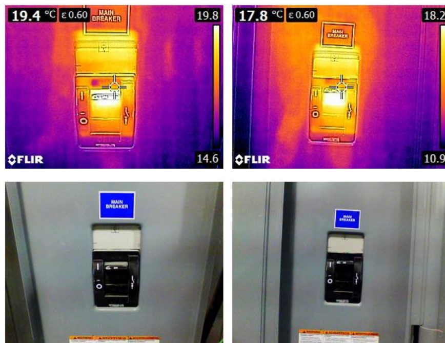
Figure 24: Temperature on the breaker at Panel CL is reduced by 1.6°C.
