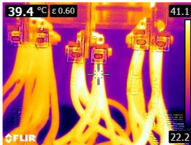
Figure 18 9-20-2018 4:38pm load on B Phase 1250 Amps Temp=39.4°C (After installation of EP Units)
