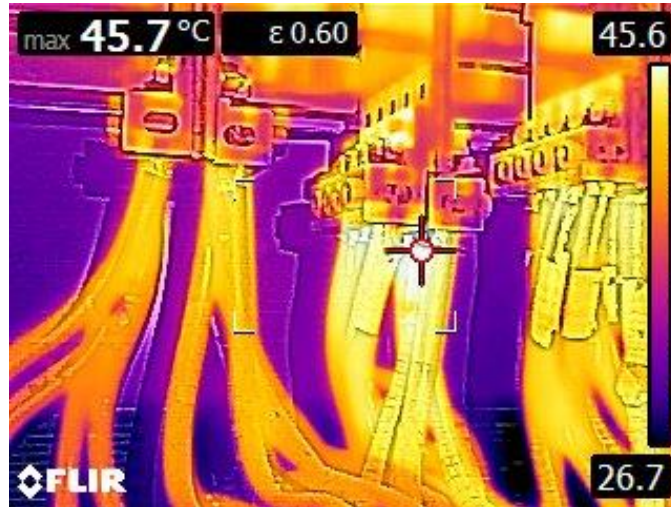
Figure 17 8-7-2018 8:16pm load on B Phase 1175 Amps Temp=45.7°C (Before installatin of EP Units)
