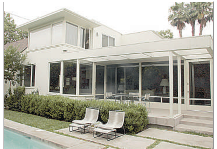
The rear of Brooke Anderson's home overlooks the pool. The house is designed around a pinwheel-shaped plan.
