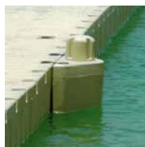
Finishing polyethylene cap
