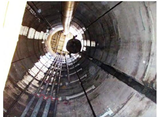
Figure 7 Looking up from shaft sink showing brattice slot cast into wall, pipe rack on wall and kibble
