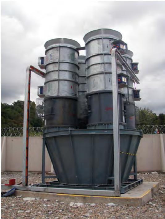
Figure 9 4 x 2 x 55 kW (110 kW) 1.250 mØ fans blowing into RB3 single 2.2 mØ intake raise on surface
