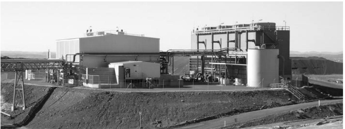
Figure 1. R67 Refrigeration plantroom (left) and 4-cell condenser cooling tower (right). Sub-stations, electrical switchroom and control room in foreground of plantroom. Pipe bridge on left supports chilled water supply and return pipes to bulk air cooler. Waste water tank in foreground of cooling tower.
