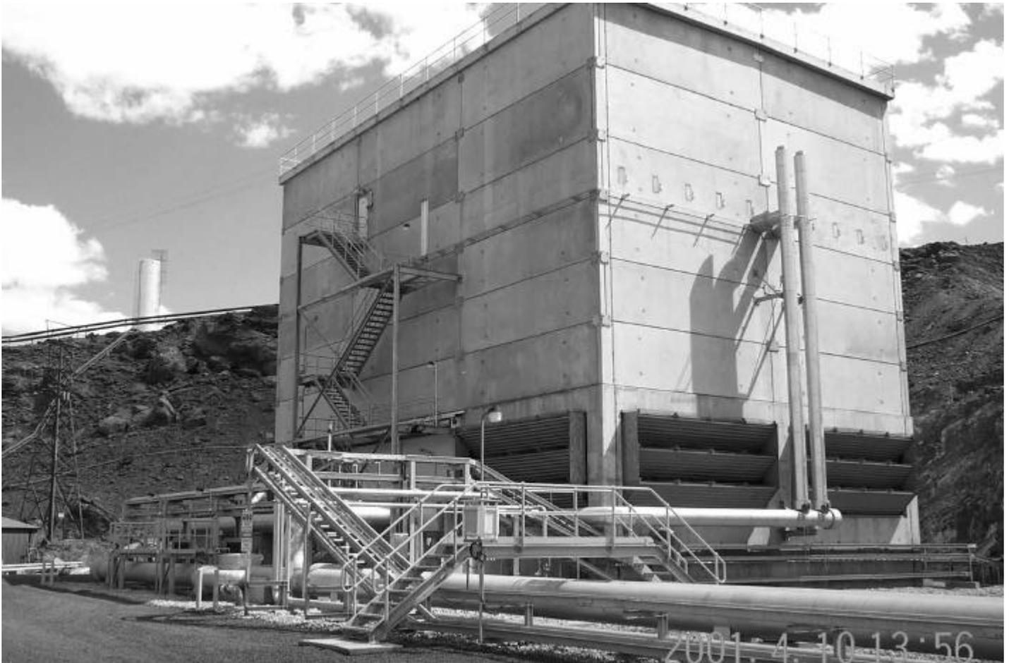
Figure 2. R67 Bulk Air Cooler (BAC). Water distribution level is about 2/3<sup>rd</sup> of the way up the BAC. Top portion of BAC is the plenum where air changes direction 180° to enter the shaft. Mid portion of plenum contains the fill where the heat exchange occurs. Bottom portion (with louvres) is the rain zone. Below the rain zone are the basins. Air enters through the louvres. The four cells surround the 7 m diameter vertical shaft.
