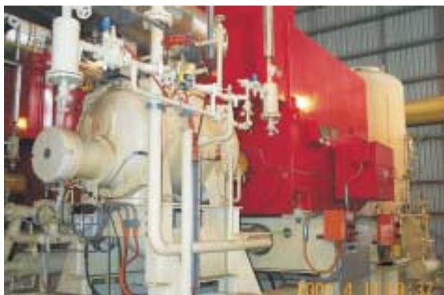
FIG 3 - Compressor (left), HV compressor motor (centre) and oil separator (right) (photo courtesy of MIM).
