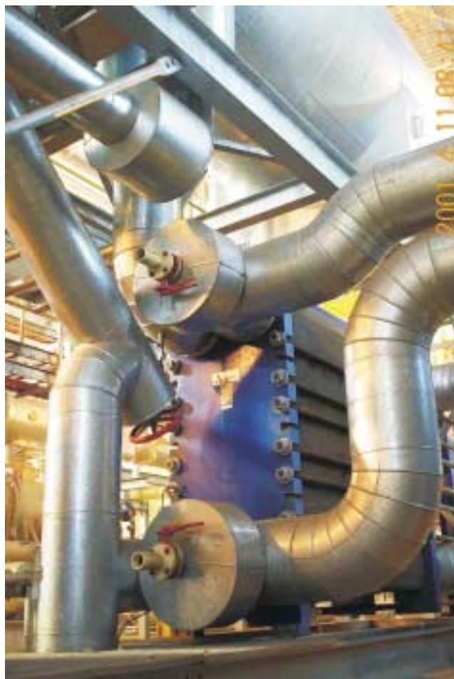
FIG 7 - Evaporator PHE with surge drum on top (photo courtesy of MIM).
