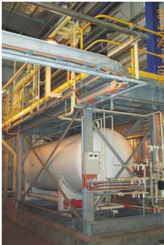
FIG 4 - Condenser PHE above (obscured) with liquid receiver below (photo courtesy of MIM).
