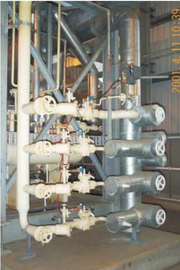
FIG 6 - Expansion valves (photo courtesy of MIM).
