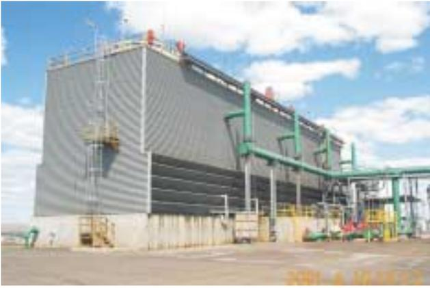
FIG 5 - Condenser cooling tower (photo courtesy of MIM).
