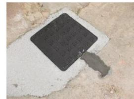
Apply a thin layer of cement or mortar on the antenna (not more than 1 cm) and close the manhole lid
