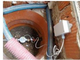
Install the HC-ANA device in the box and connect the antenna cable once it has passed through the exit hole of the made manhole. Connect the flat antenna
