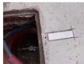
Use a piece of plastic gutter to protect the antenna. Make a recess in the ground
