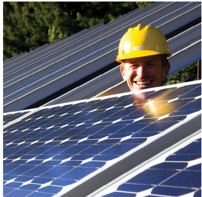
Installing solar panels, Oregon Department of Transportation.
