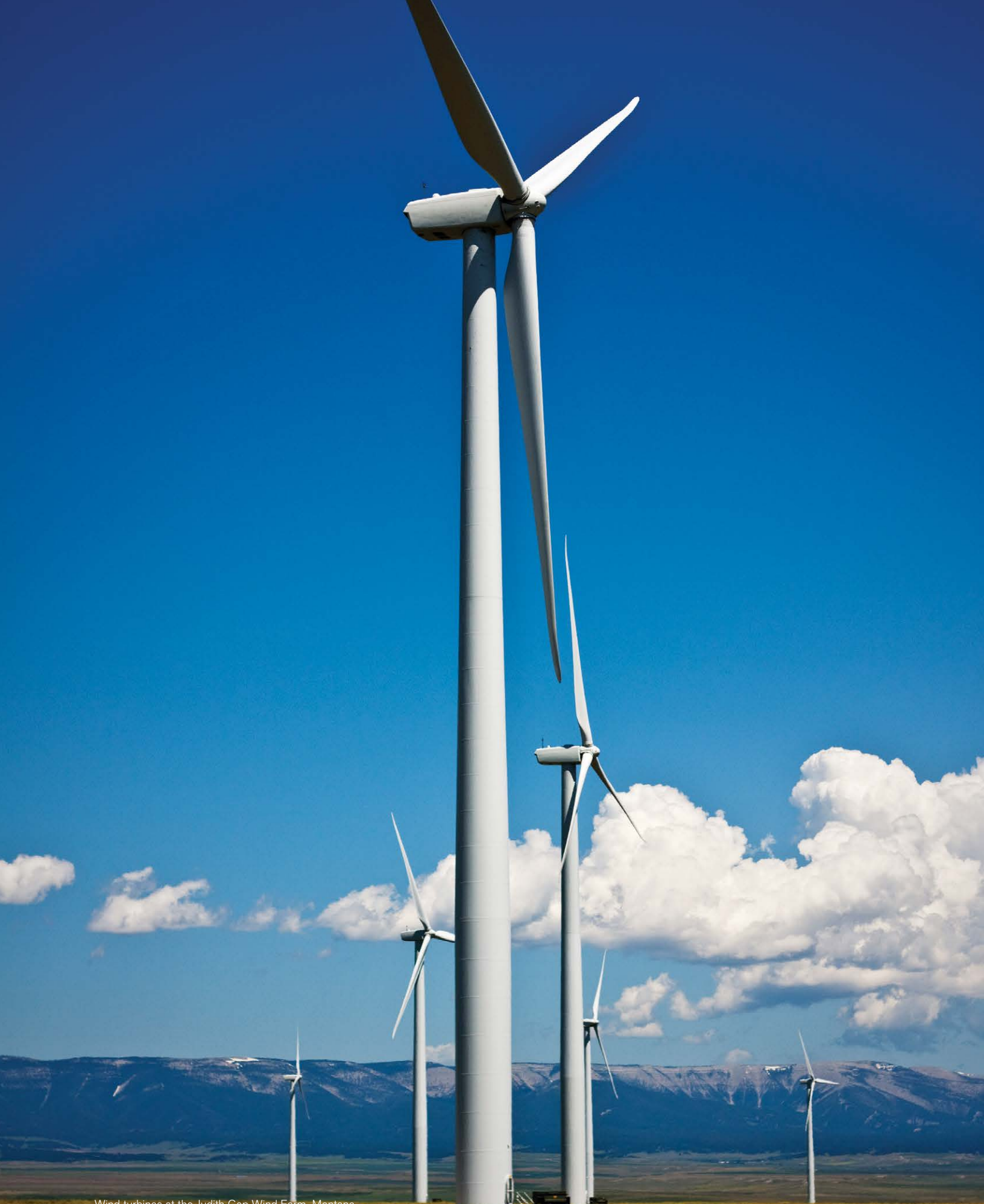
Wind turbines at the Judith Gap Wind Farm, Montana. Photo credit: Nomadic Lass
