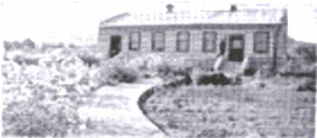
Brooklyn Cottage Hospital - 1914
