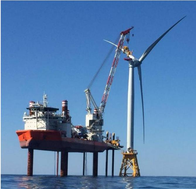
**FIGURE 1: MV BRAVE TERN INSTALLS A TURBINE BLADE AT BIWF, (PHOTO: DEEPWATER WIND, LLC)**
