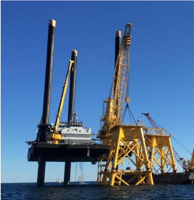
**FIGURE 6: LIFTBOAT LB ROBERT INSTALLING A WTG FOUNDATION JACKET AT BIWF (PHOTO MONTCO OFFSHORE)**
