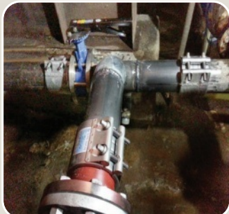
▲ Netherlands desalination treatment facilities
