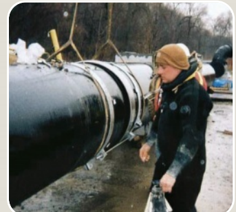
▲ UK: district heating work
