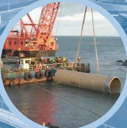
Installation of ocean bed blocks
