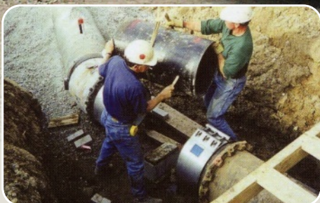
▲ Repair work for pipes replaced underground
