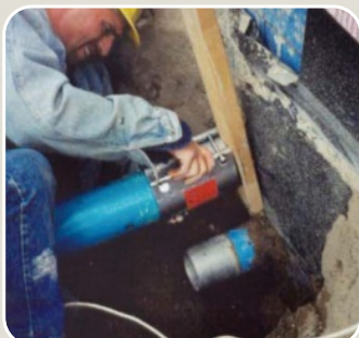
▲ U.S.: sewerage repair work
