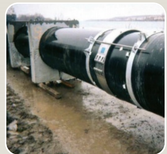
▲ U.S.: nuclear power plant
