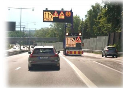
Road Works Warning
