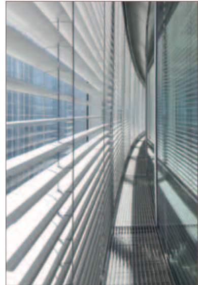
The ladder braid attached to the omega punching ensures correct spacing between the slats.
