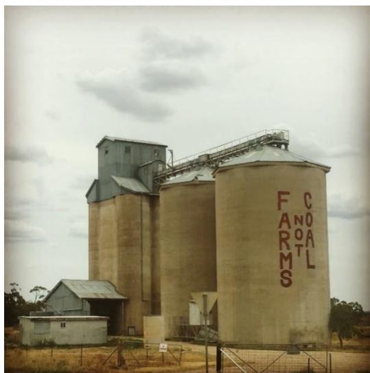
Figure 3. Silo, Liverpool Plains, NSW
