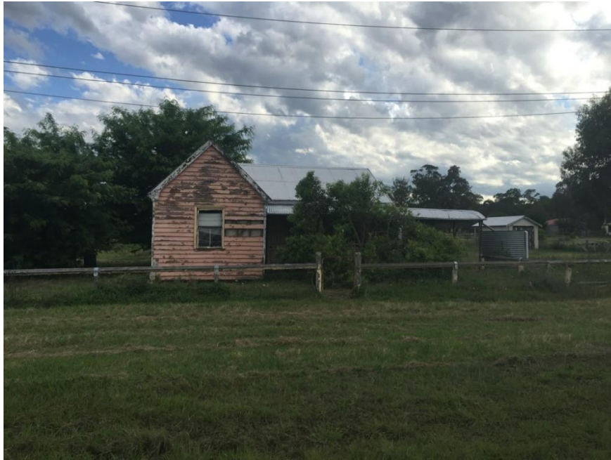
Figure 2. Houses left behind, Wollar
